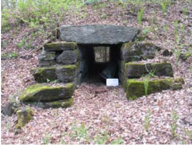
A prime example of a hidden gem along the LVRT, a cattle pass from long ago
