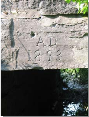
Dated box culvert on the LVRT
