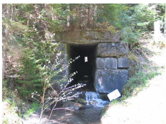
"A box culvert along the LVRT"
